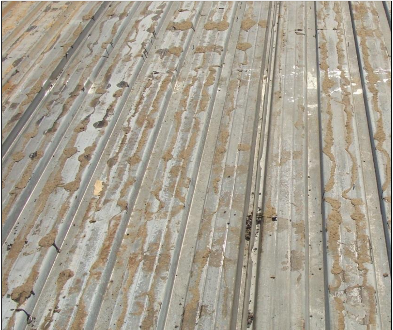
Photo of Level 1: No Visible Corrosion
